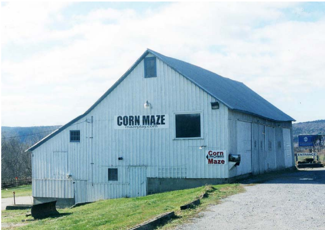
Figure 6. View of the threshing barn (Connie Kheel photo).
