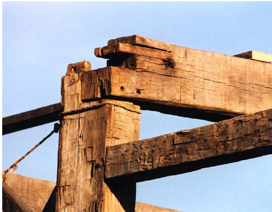
Figure 12. View of a typical joint during the restoration of the barn. Note the marriage marks incorporating a circle and slashes of the race knife, just below the lower part of the joint (Photo courtesy Connie Kheel).
