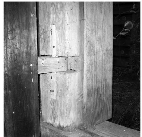
*At near end wall of Wemple barn is wagon door post with slot for wooden hinged door. Door that swings on wood pintle is open and has swung into the barn.*
