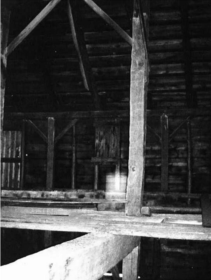
View of H-frame with long post in three-bay three-aisle barn at the Oliver homestead. Very long 15½' *verdieping* of H-frame. Note short purlin brace at top of post.
