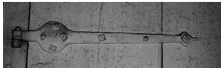
Handforged iron hinges with round nailing pad.
