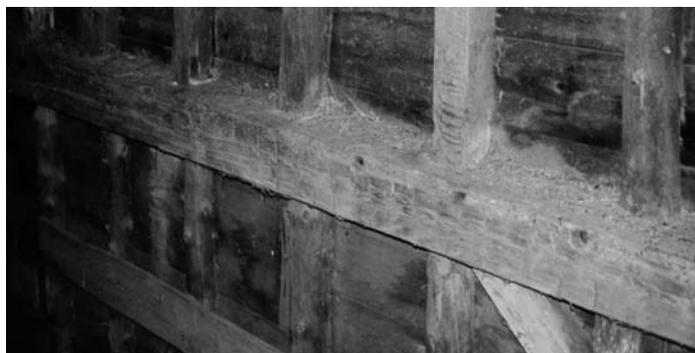
*View of recycled hay-barrack post at north end wall in bent in three-bay three-aisle barn at the Oliver homestead. Note holes at corner of post that functioned in raising and lowering of adjustable roof in former hay barrack. Round pole studs appear above and below the post.*
