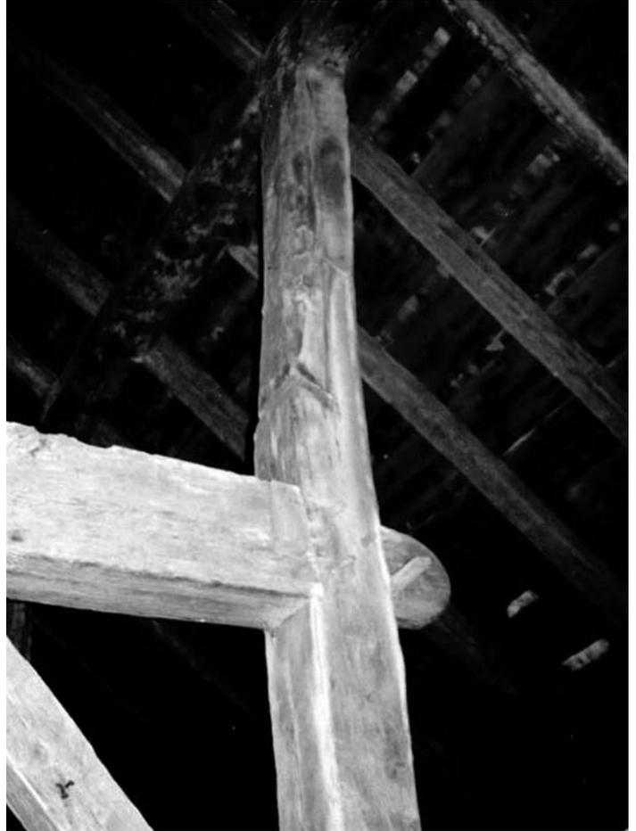
View of H-frame post that was later spliced circa 1830 in four-bay three-aisle classic barn at the Oliver homestead. Note hewn rafters in common rafter system in roof.
