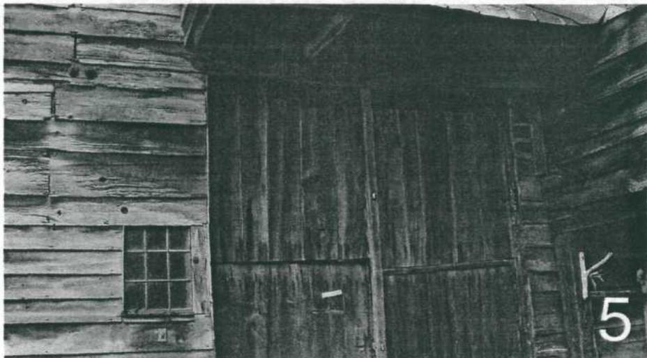
Seen are original wooden hinged single height doors at last interior H-frame in Bogart U-barn in Marletown, Ulster County, New York. Doors lead into the last bay, full of dirt. At sides of both door posts are remnant horizontal sheathing.
