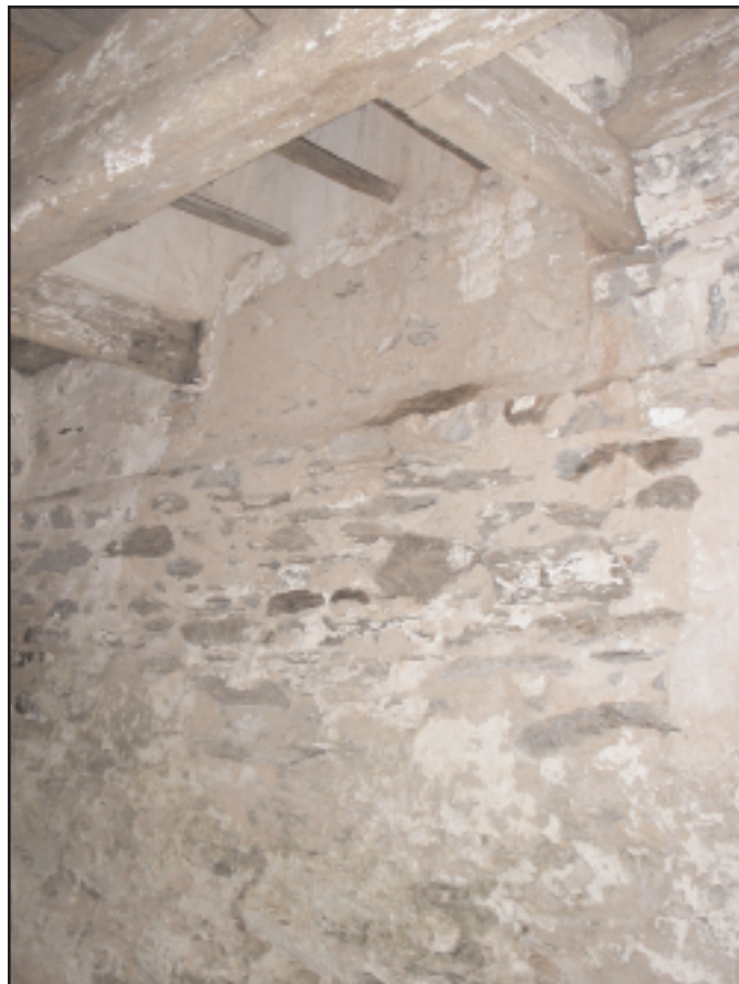
Photo 3. The jambless fireplace in the Beatty-Cramer spring house.
