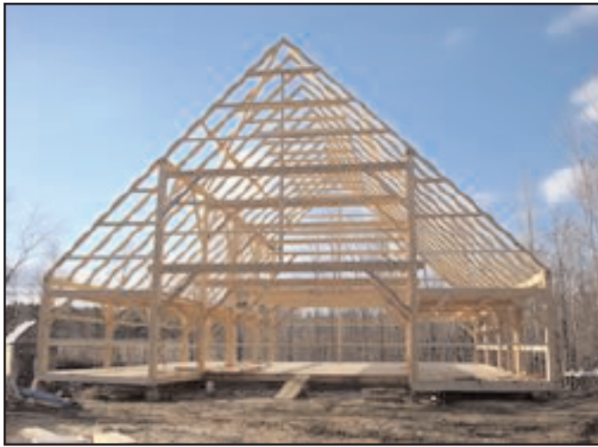
Photo 2. The completed frame.
