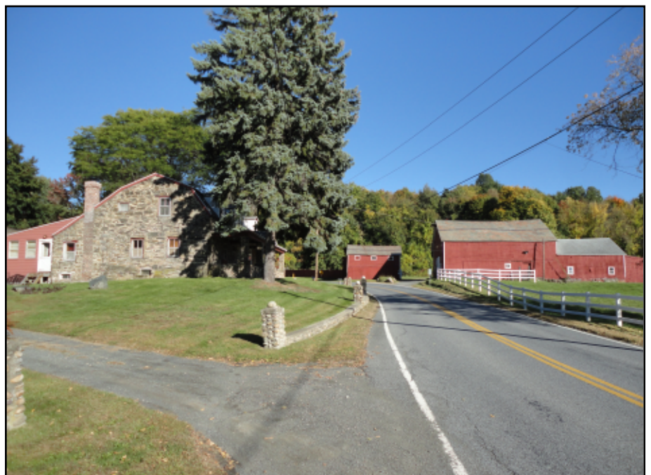
Photo 2. View looking east showing relationship of house, single aisle barn and New World Dutch barn (October 2015).
