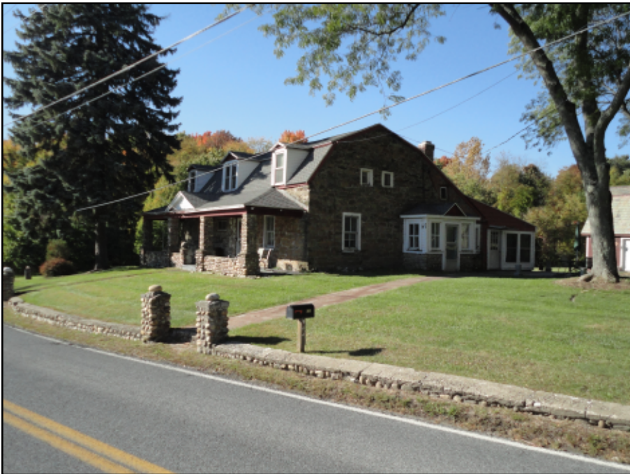
Photo 3. View looking northwest at the Beam-Dusenbury house (October 2015)
