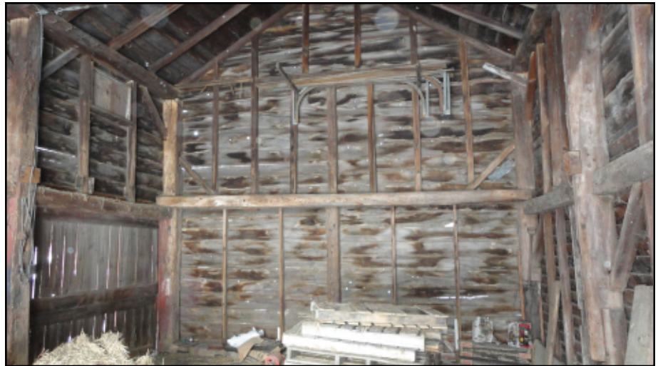
Photo 10. Interior view looking north in the single aisle barn (January 2011).
