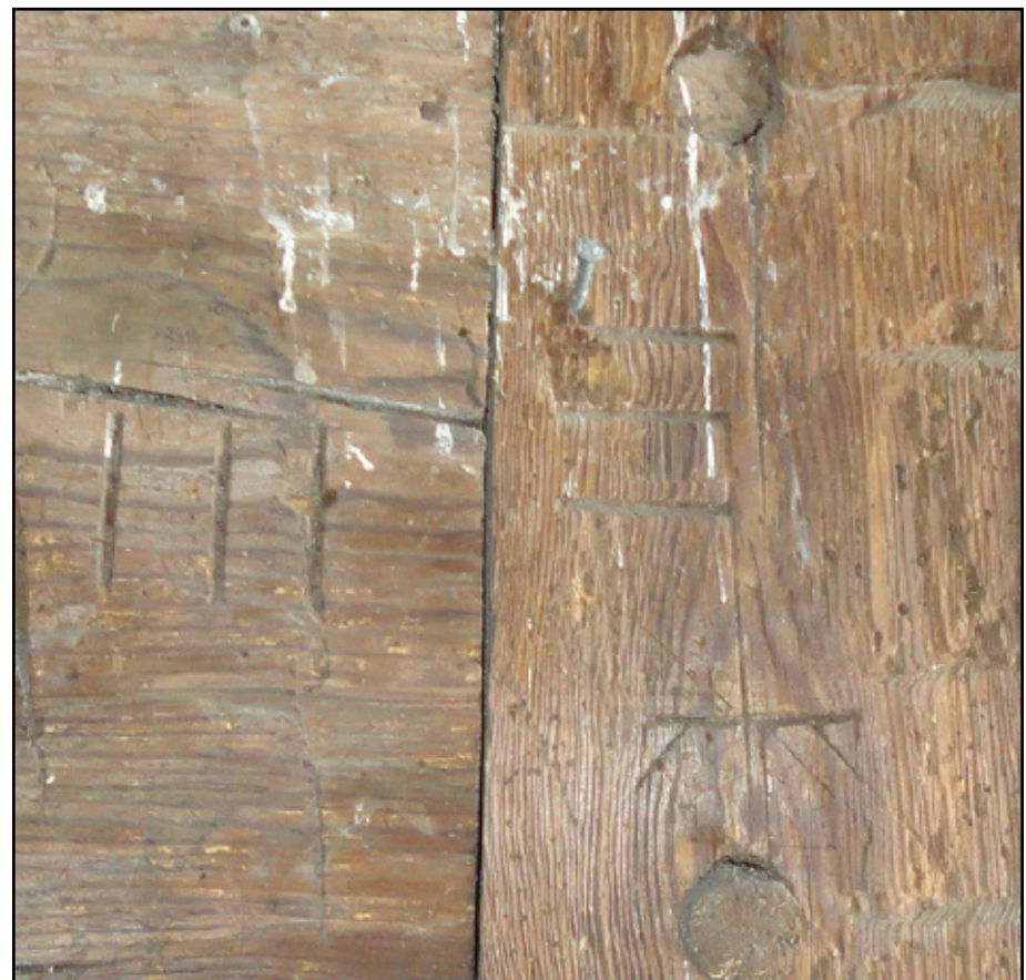
Photo 7. Detail showing inscribed drawing on face of east bent post 3, together with marriage marks (January 2011).
