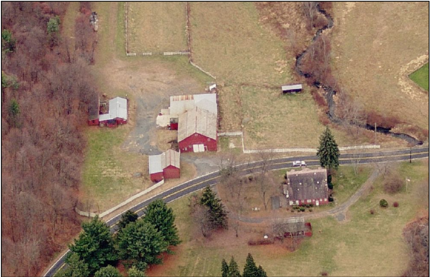
Photo 1. Aerial view looking south, showing the relationship of the house, barns and landscape features including the Piscawen Kill (n.d., c.2011).
