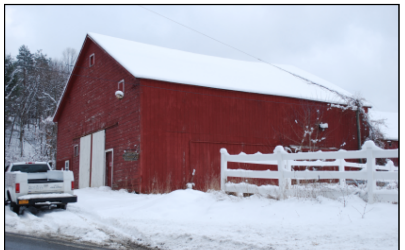
Photo 1. The Beam-Dusenbury New World Dutch barn (January 2011).
