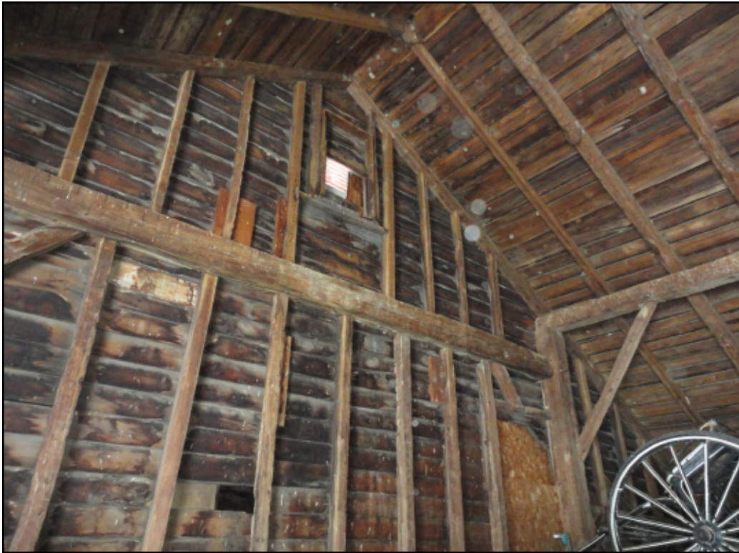
Photo 8. Interior of barn, looking south-southwest from the loft (January 2011).
