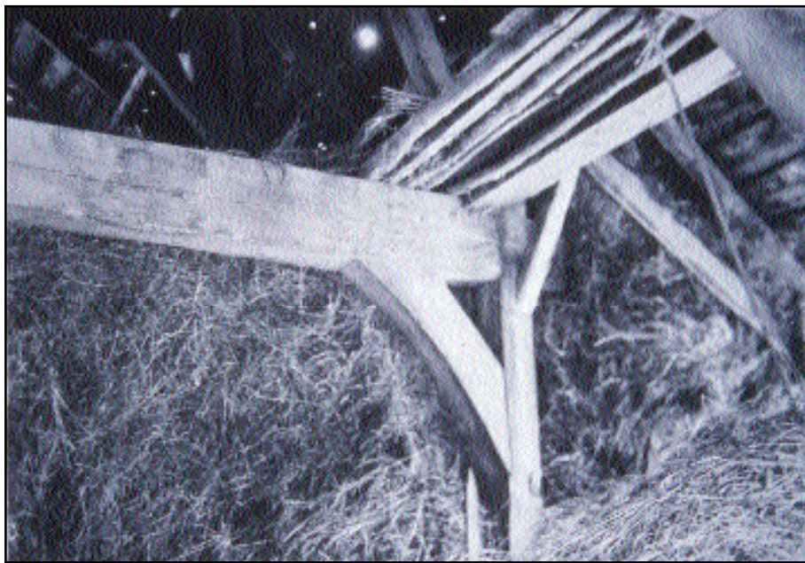
Photo 2. Van Bergen barn. About 1680, only a decade after the barn in the 1669 contract of Jeremias van Rensselaer was erected, another early Dutch barn was put up at Leeds in present-day Greene County, New York for Marte Gerrit van Bergen, a resident of Rensselaerswijck. The building collapsed in the 1970s. This rare view of its seventeenth-century interior shows anchor beams, posts, and the curved soffit of a brace, with saplings above (Photo of unknown date by Vincent Schaefer, from his 1994 book, Dutch Barns of New York, An Introduction , (Purple Mountain Press), reproduced with permission.)
