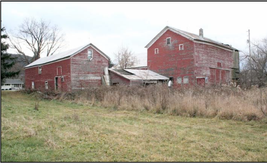
Photo 4. English barn and cow stable #1 at the Shafer farm Dutch barn complex, facing southwest, December 2009 (Photo by the author).
