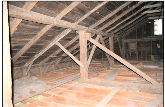
Photo 3. Interior of Dutch barn showing rafters, H-bent post, anchor beam, cut-off transverse tie-beam, longitudinal sway bracing, and modern bracing, facing southeast, December 2009 (Photo by the author).
