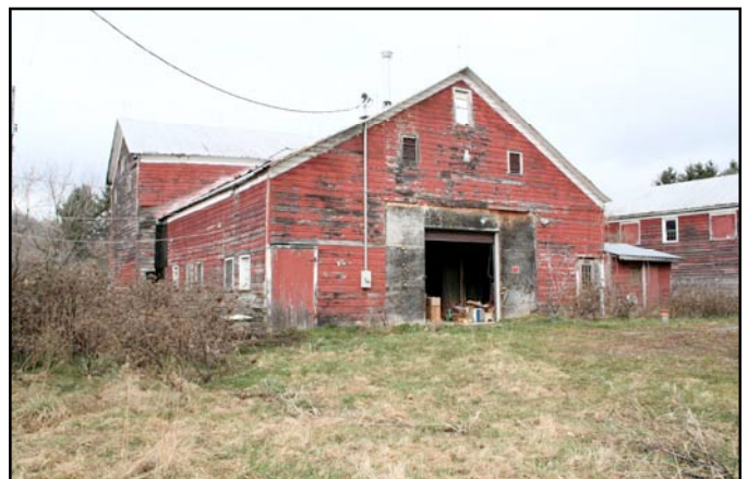
Photo 2. The Shafer New World Dutch barn anchored a complex of four barns on the north side of NYS Route 7 near Warnerville; view facing northeast, December 2009 (Photo by the author).
