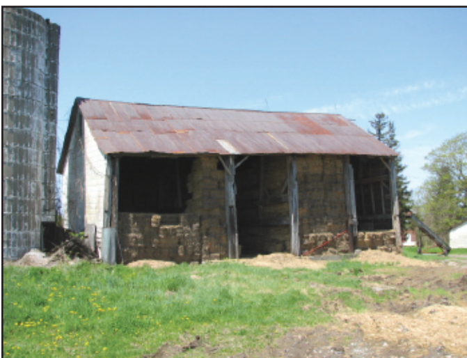
Photo 7. Swing-beam barn, looking west-northwest, May 2007 (Photo by W. Wheeler).
