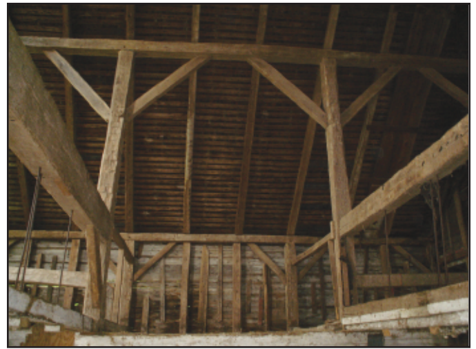
Photo 4. Bents B and C, looking west, May 2006.
