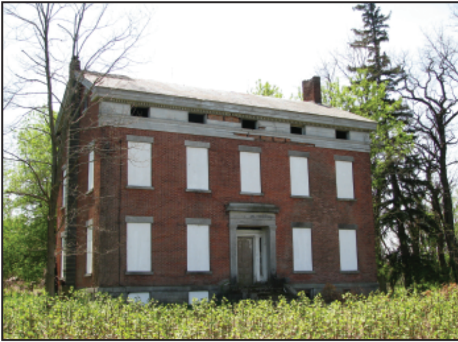
Photo 10. View of front of house, looking south-southwest, May 2007 (Photo by W. Wheeler).
