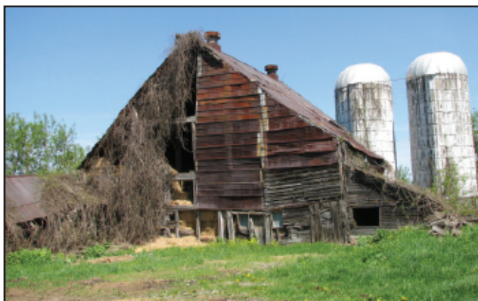
Photo 2. The Dutch barn, looking north-northwest, May 2007 (Photo by W. Wheeler).
