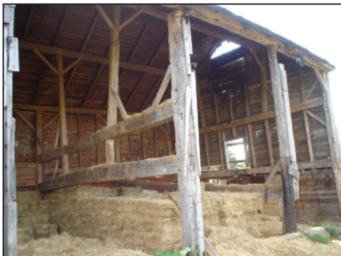
Photo 8. Detail showing swing beam with double tenon connection to post, May 2006.
