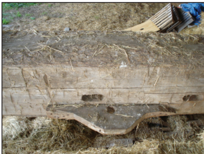
Photo 9. Detail showing attachment on swing-beam for threshing pole, May 2006.
