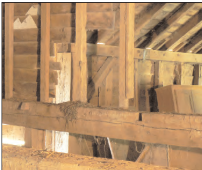
Photo 11. Details of the end anchor beams. At the front end you can see the end of one of the pence support beams is still in place.
