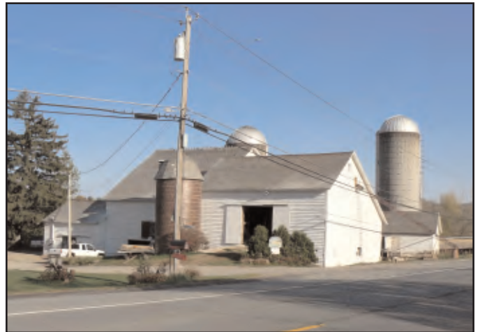
Photo 2. The barns seen from the southwest. The Dutch barn is behind the 1916 tile silo. The barn closest to the road dates to the later nineteenth century.
