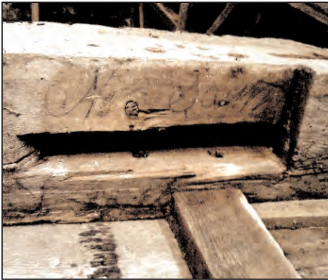
Photo 1. Reused post with "No 3 South" inscribed on its face (L. Lawler).
