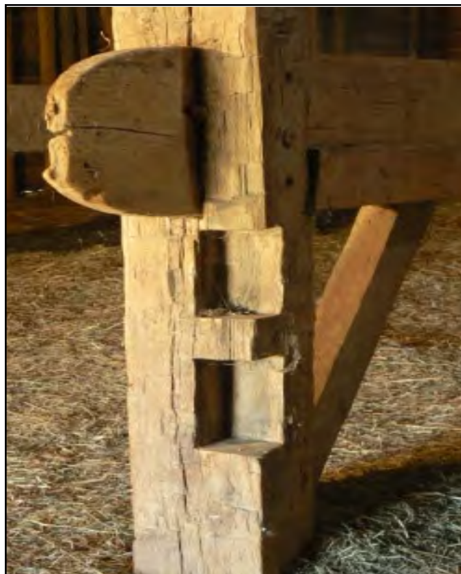
Photo 10. The open mortises cut into the face of the post seen here may have held the supports for the ramp.
