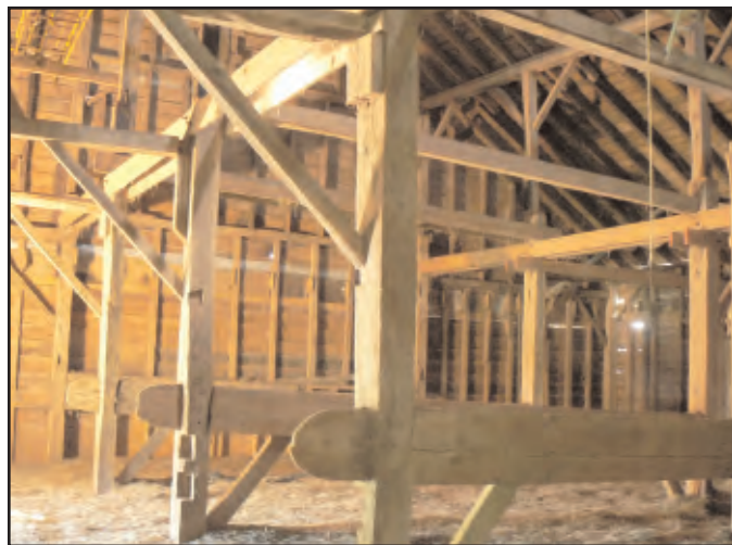
Photo 7. Interior view of barn, showing later framing.
