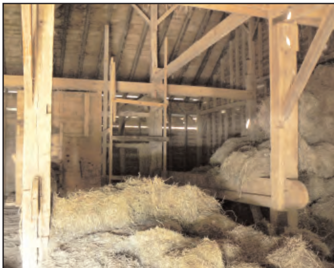
Photo 9. The anchor beams are both pegged and wedged. Unusually, the anchor beam tenons are centered on the posts, as seen in this view. Note the cutouts in the anchor beams, forming a ledge which held the floor of the second level. This detail can also be seen in Photo 10.
