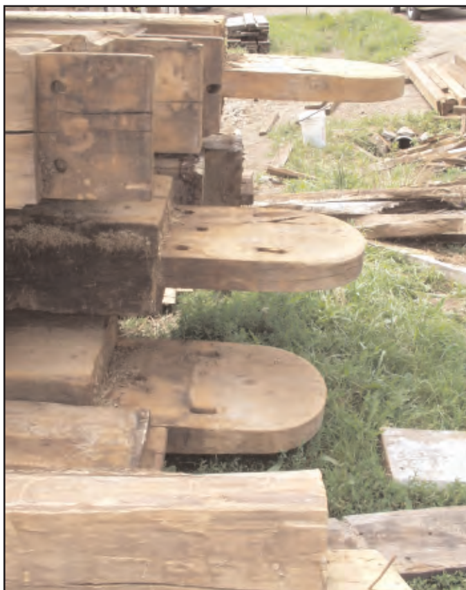
Photo 3. The anchor beams.
