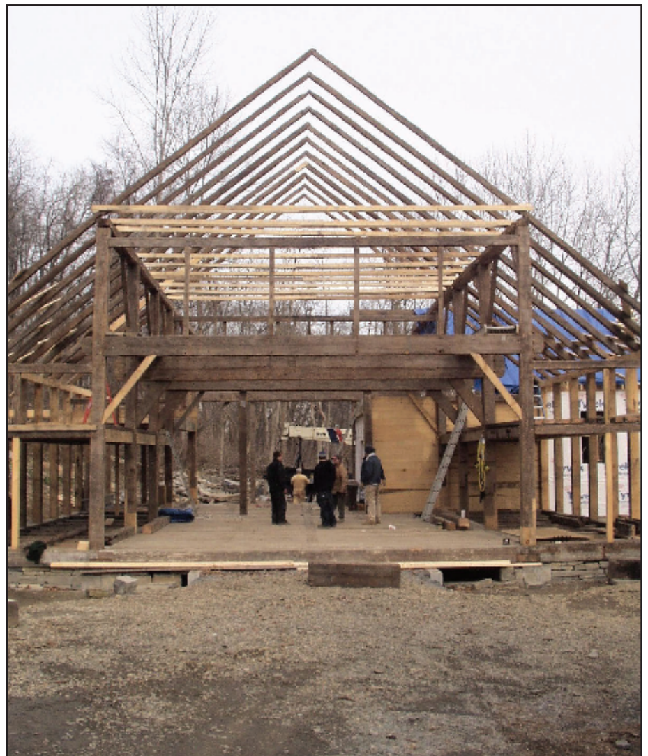
Photo 4. River Street barn on its new site, November 2009. Old rafters are up on the 3-bay section. Partial siding on 'interior' gable wall that will separate the barn from the workshop (Photo by Keith Cramer).
