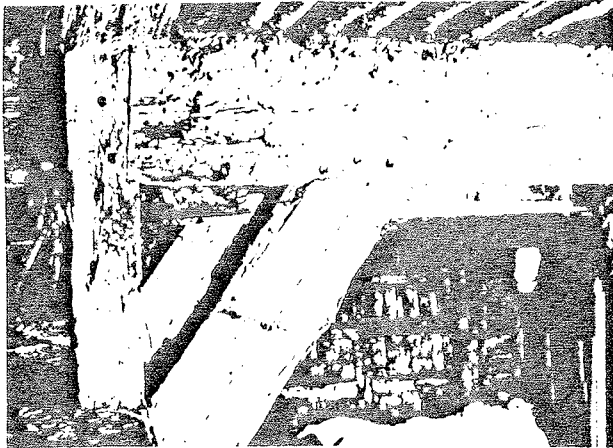
Anchor Beams + Braces
