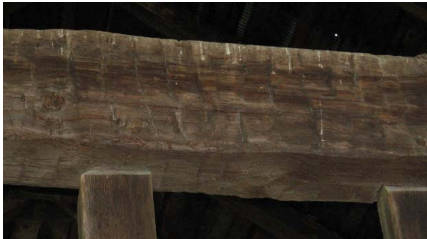
Figure 1. The surface of this beam clearly indicates that it was hand-hewn rather than sawn.
