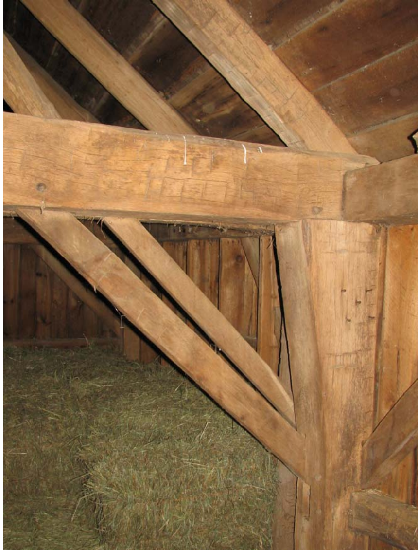
Figure 5. Typical joint in the O'Donnell Hill barn. The flared top of the "gunstock" post is particularly evident in this shot.
