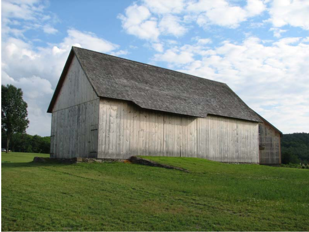
Figure 11. View of the tying joint barn at Nipmoose.
