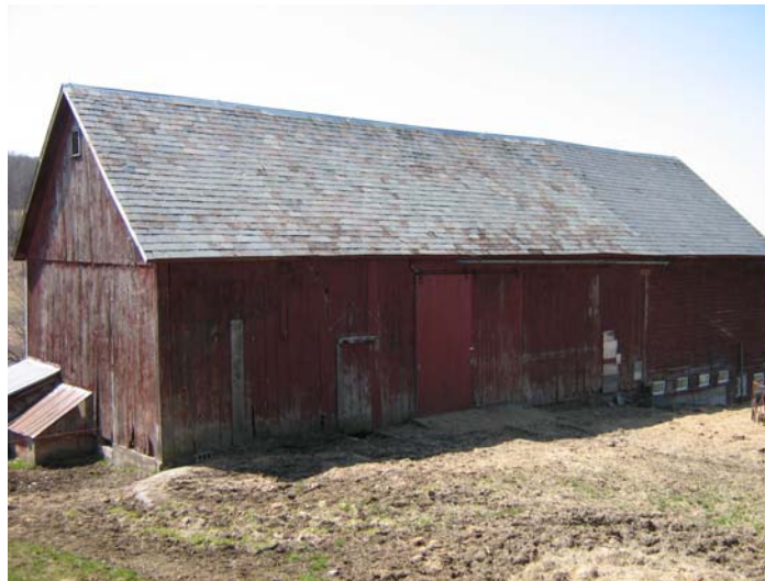
Figure 4. View of the three-bay threshing barn, with later one-bay addition to the right, on the O’Donnell Hill farm, Town of Jackson.
